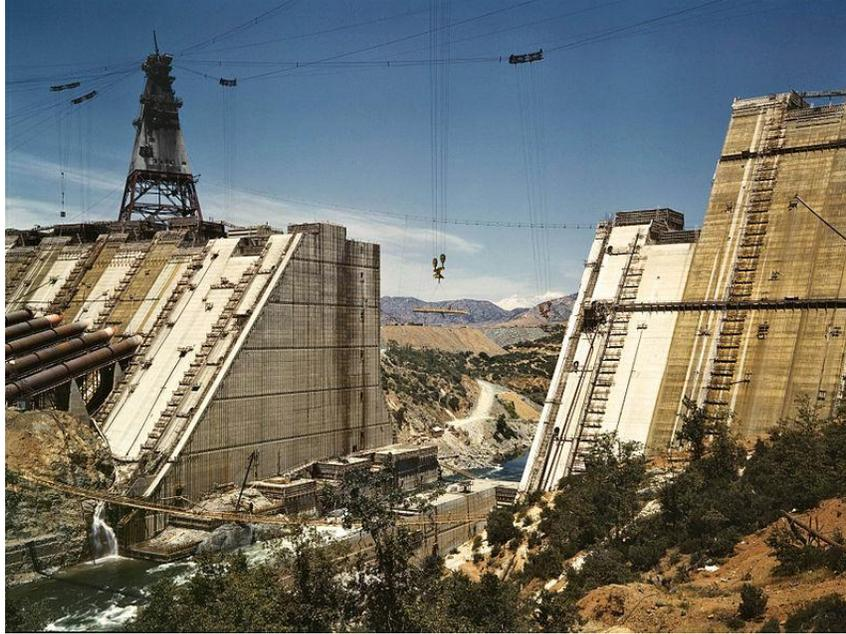
Shasta Dam is one of the largest dams in the United States. The dam is 602 feet tall and 883 feet thick at its base. Located in Northern California, it blocks the flow of California's biggest river, the Sacramento River. This dam forms a big lake behind it, Lake Shasta, which has a 365-mile-long shore line.
